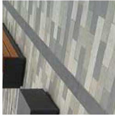
Block Paving - Type E Material: Permeable Concrete Block Colour: Midnight Grey Unit Size: 200 x 100 Pattern: Linear
