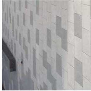
Flag Paving - Type A Material: Concrete Flag Colour: Mixed Shades (Light/ Medium Grey) Unit Size: 300 x 200 Pattern: Stretcher Bond
